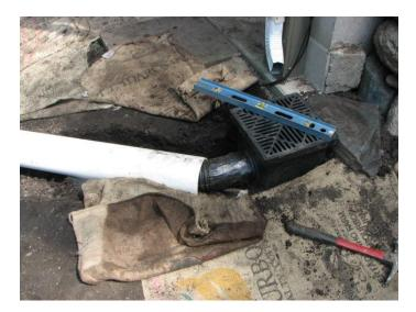
A catch-basin with grate (generally no smaller than 12 in x 12 in) should be set in level beneath a downspout. Water is then directed through drain tile underground.
