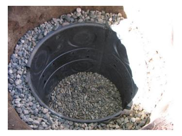
Routinely (weekly) check the inlet for debris or accumulated sediment that may block water flow. Remove accumulated debris and litter, especially around inlet and outlet areas.
