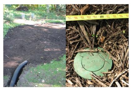
On the left is a drain-tile installation ending in a raingarden. The outlet end will have a screened attachment or a pop-up (pictured on the right) to prevent mulch or animals from entering.
