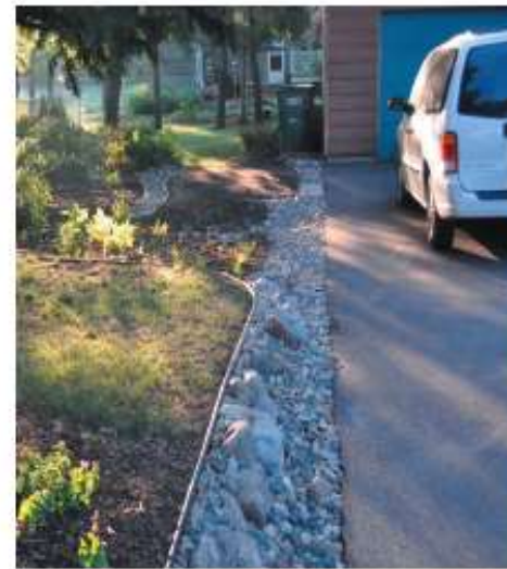
BOTTOM RIGHT: DRY CREEK ALLOWED WATER TO EXIT DRIVEWAY AND ENTER A RAINGARDEN
