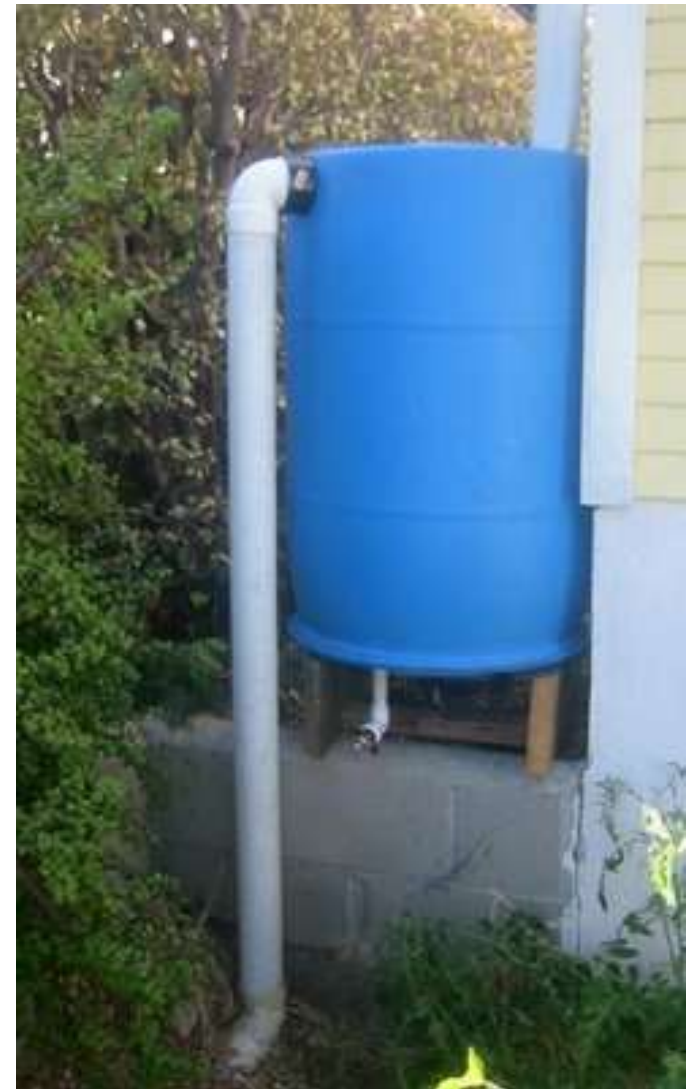
Rain barrel is placed high & overflow is properly sized.
