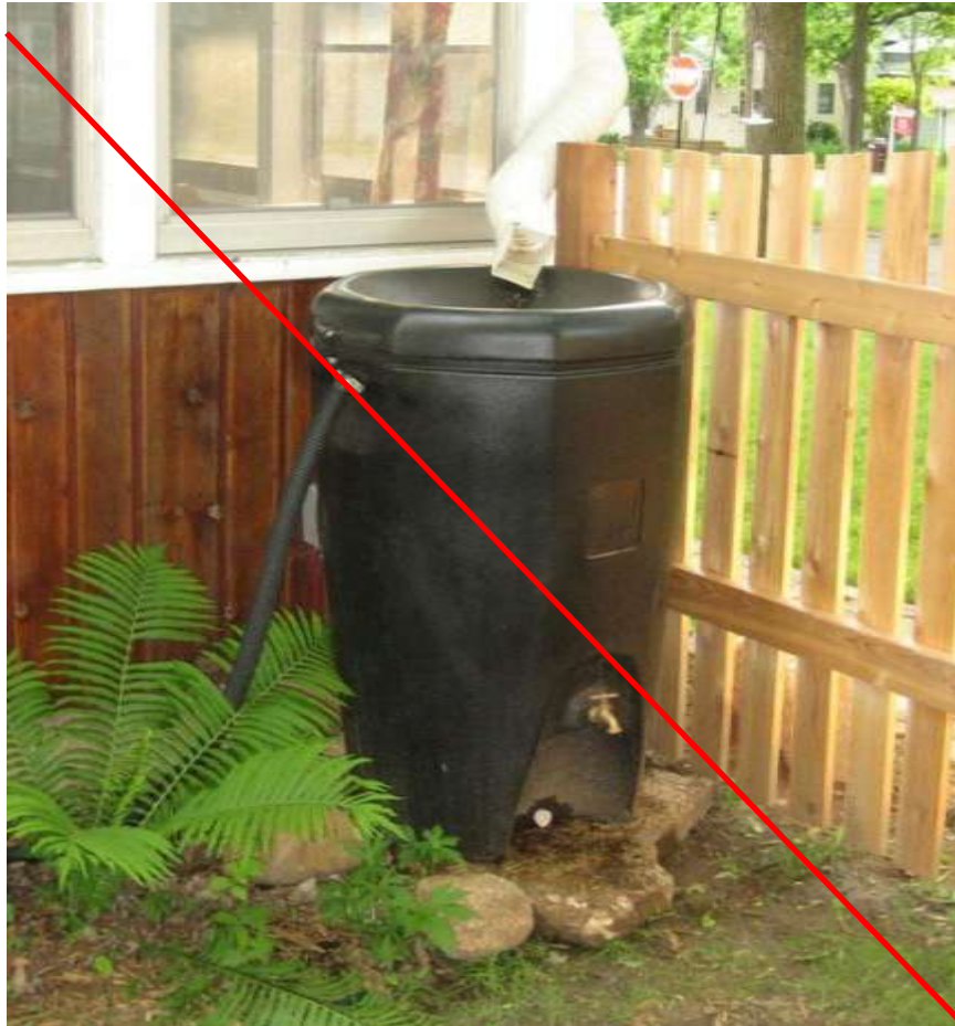
Rain barrel is too low to the ground & the overflow too small.
