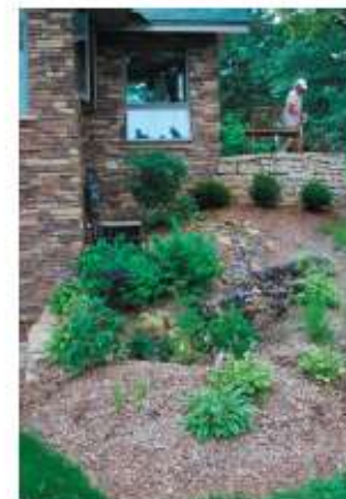
TOP RIGHT: DRY CREEK CATCHES ROOF RUNOFF AND DIRECTS WATER TO A RAINGARDEN
