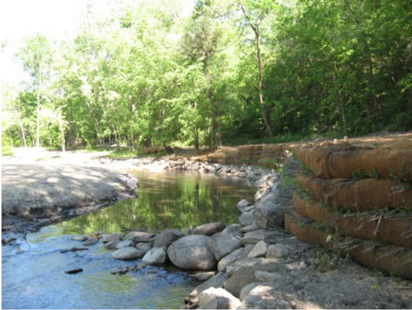
Figure 7. Bioengineered streamline stabilization along Minnehaha Creek in Minnehaha Falls Park in Minneapolis.
