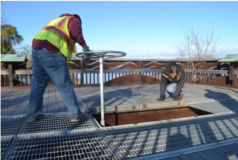
Figure 4. Closing the Grays Bay dam.
