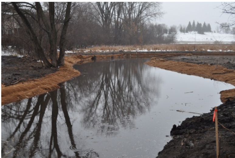
Figure 5. Restoration work in progress along Reach 20 of Minnehaha Creek
